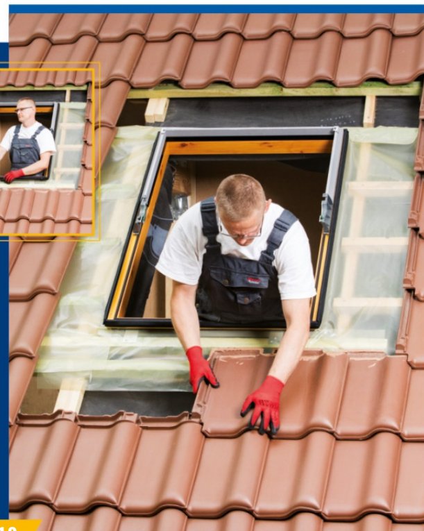
Arrange the lower row of the chamfered roof tiles.
