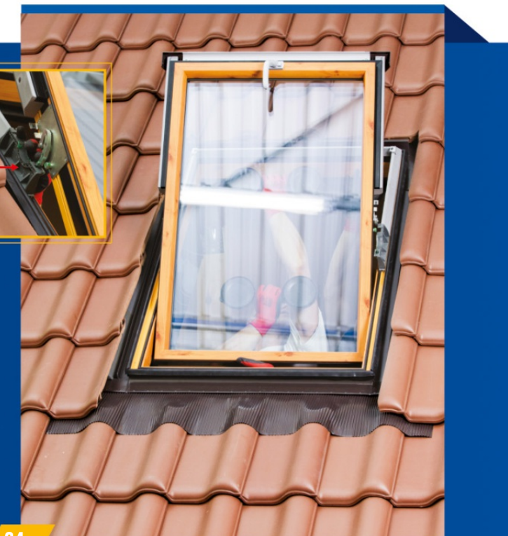
Install the leaf in the window frame as shown in the photos.
