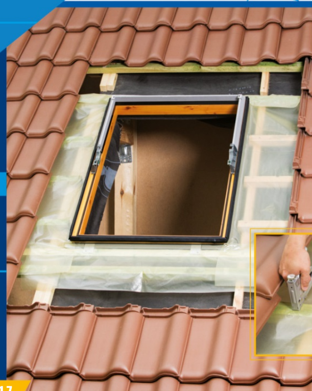
Installation of roof membrane or / and flashing made of vapour permeable membrane.
