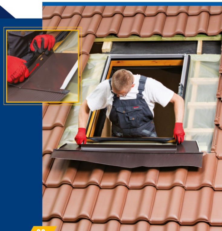
Install the lower element of the sealing flange by sliding the flange onto the screw fixed on the frame.
