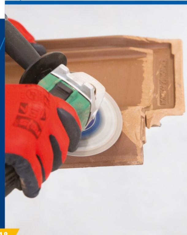
Chamfer the lower row of roof tiles at an angle of 45° (under the flexible element of the flange).
