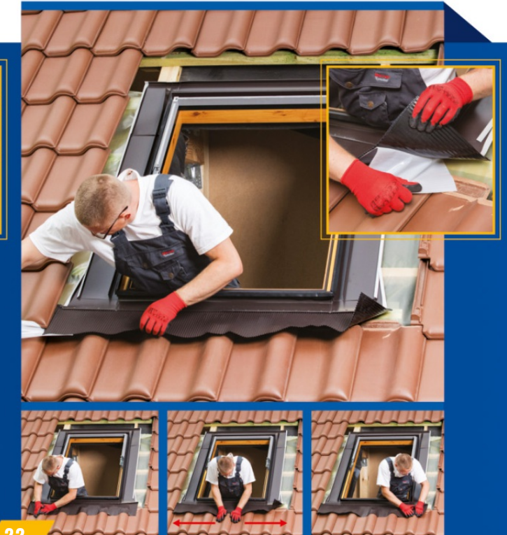
Glue the flexible cover flashing to the roof tile. Tear off the protective tape and glue the cover flashing, beginning from the middle and keep profiling it so that it clings well to the roof tile.
