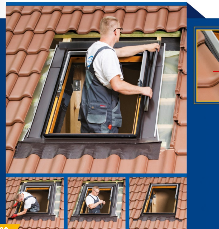
Install sealing wedges on the flange on the upper and side elements and arrange the roof tiles. Cut the roof tiles if necessary to adapt them to the flange.
