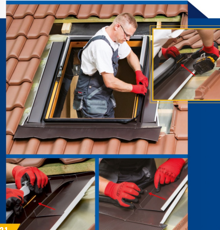
Install the flange elements using the screws fastened in the window frame. Proceed in this order: left-side and right-side element, then upper element. Once the elements are secured and adjusted, tighten the screw used to fasten the flange.
